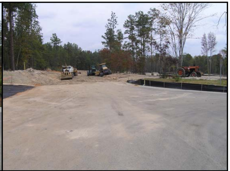
Looking towards phase 2 from Rice Creek Farms Rd.
